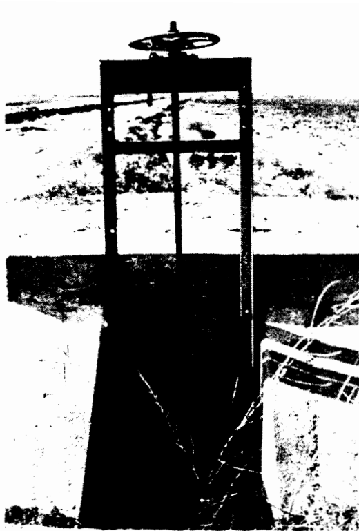
Figure 8.4 Two typical slide gates for surface irrigation systems. (a) Screw gate from central Utah. (b) Trapezoidal jack gate. (Courtesy of Dr. G. E. Stringham.)
